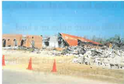
A local school destroyed by the storm surge.
