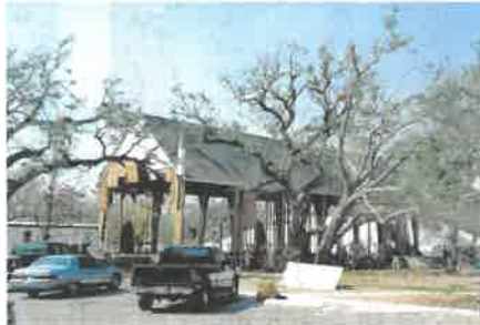
This is a church whose walls were destroyed by the storm surge.
